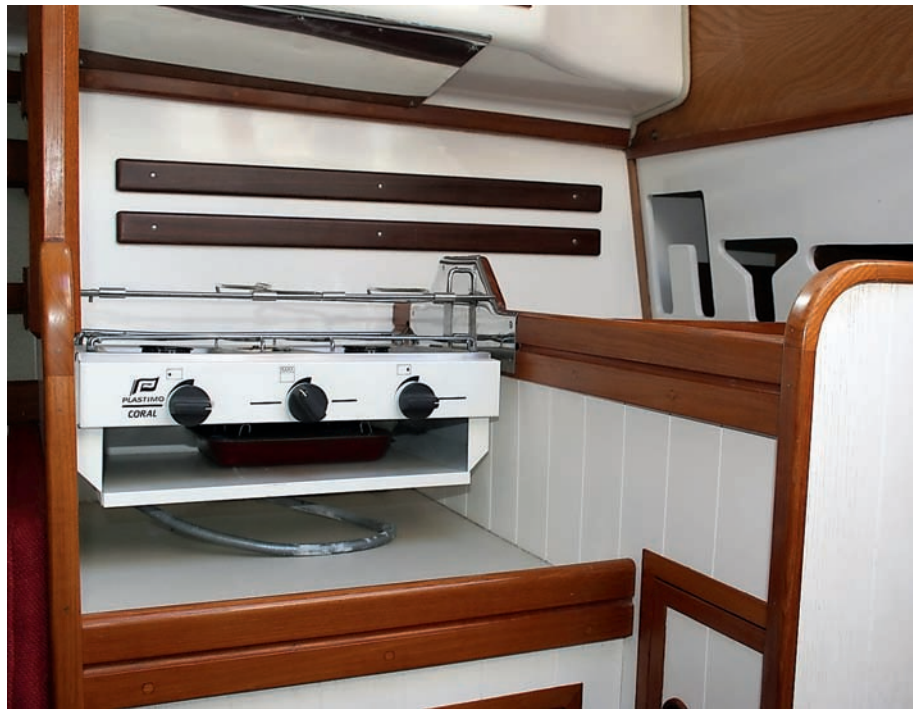
The standard galley with gimballed two burner and grill unit.
